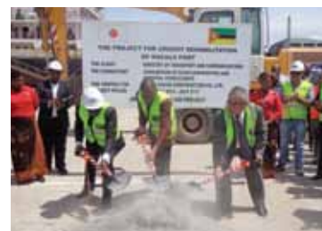
Nacala Port Rehabilitation
