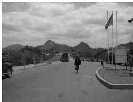
Photo-2 Around the gate
