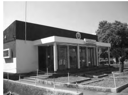
Photo-1 Border main office
