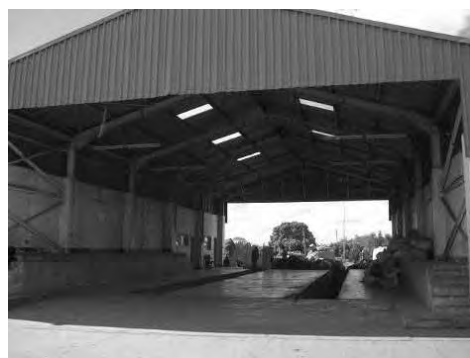
Photo-2 Inspection facility
