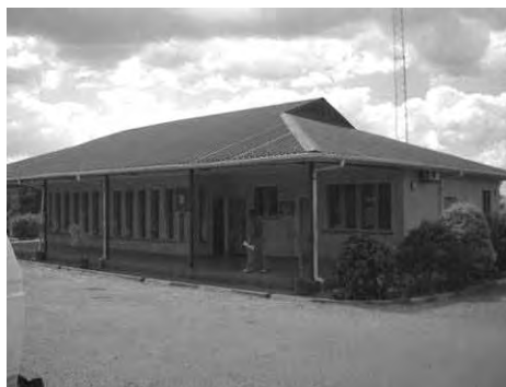
Photo-1 Border post main office
