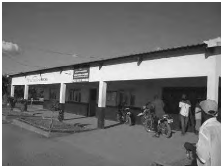
Photo-1 Border post main office
