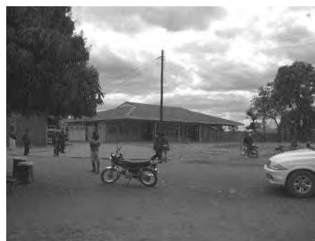
Photo-2 Border post main office
